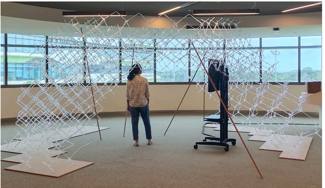
Student team A designed a non-orthogonal lattice structure ( virtual version above), while team B constructed it using the AR app given to them by that team (completed structure below).
