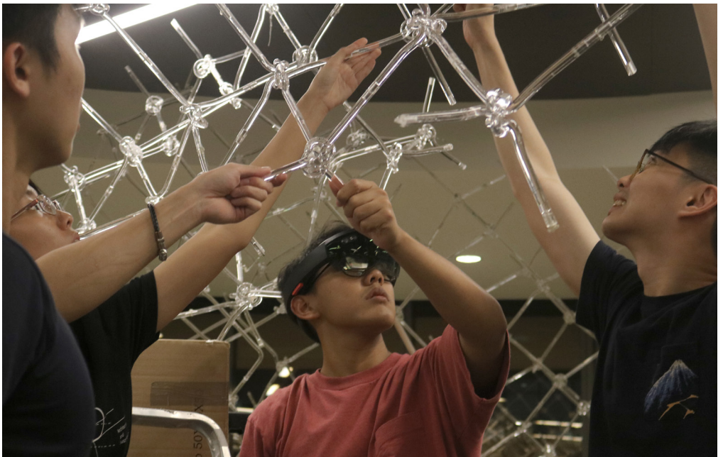
Students used the AR apps they developed to display holograms of the structures in incremental states on the HoloLens, then assembled physical modules to match the virtual reference.
